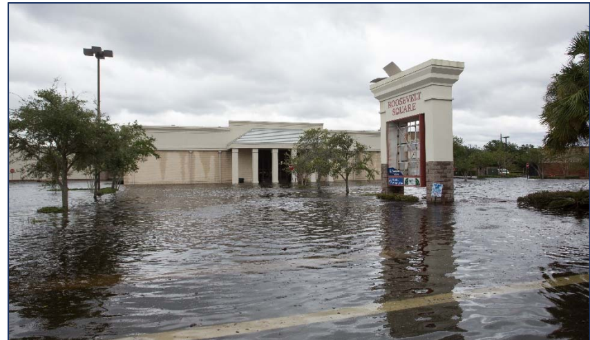
Hurricane Irma – Roosevelt Square Shopping Center, September 11, 2017
