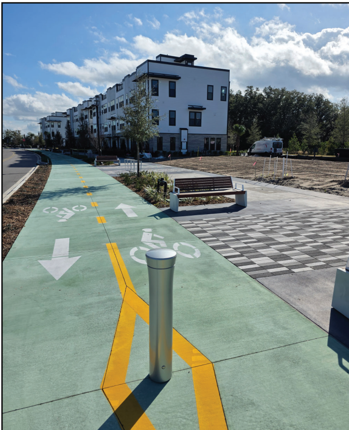
State of the Art: The RiversEdge community boasts a protected two-way cycletrack tinted a bright green, with ample pedestrian space, seating, and bicycle parking. RiversEdge construction incorporates many cutting-edge active transportation design standards.
