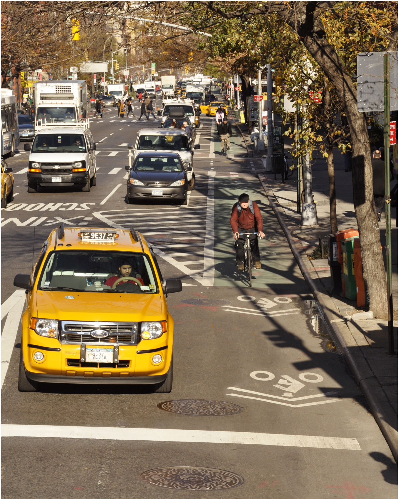
A mixing zone along New York City's 2nd Avenue separated bike lane. (Source: NYC DOT)
