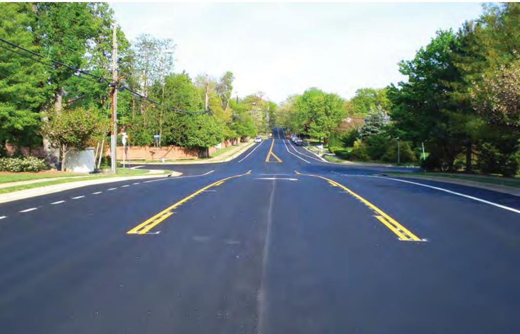
Figure 23. Transition from 3-lane to 2-lane Cross Section, Oak Street, Merrifield, VA Photo Credit: Virginia DOT
