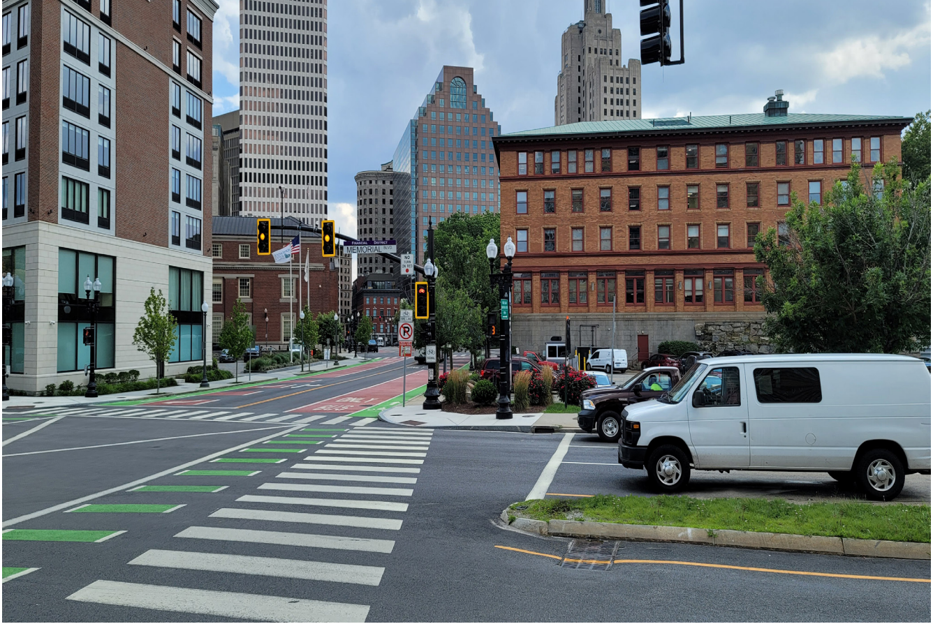
Figure 3. Signalized intersection with bicycle lanes, wide crosswalks, and bicycle signal face. Source: FHWA.
