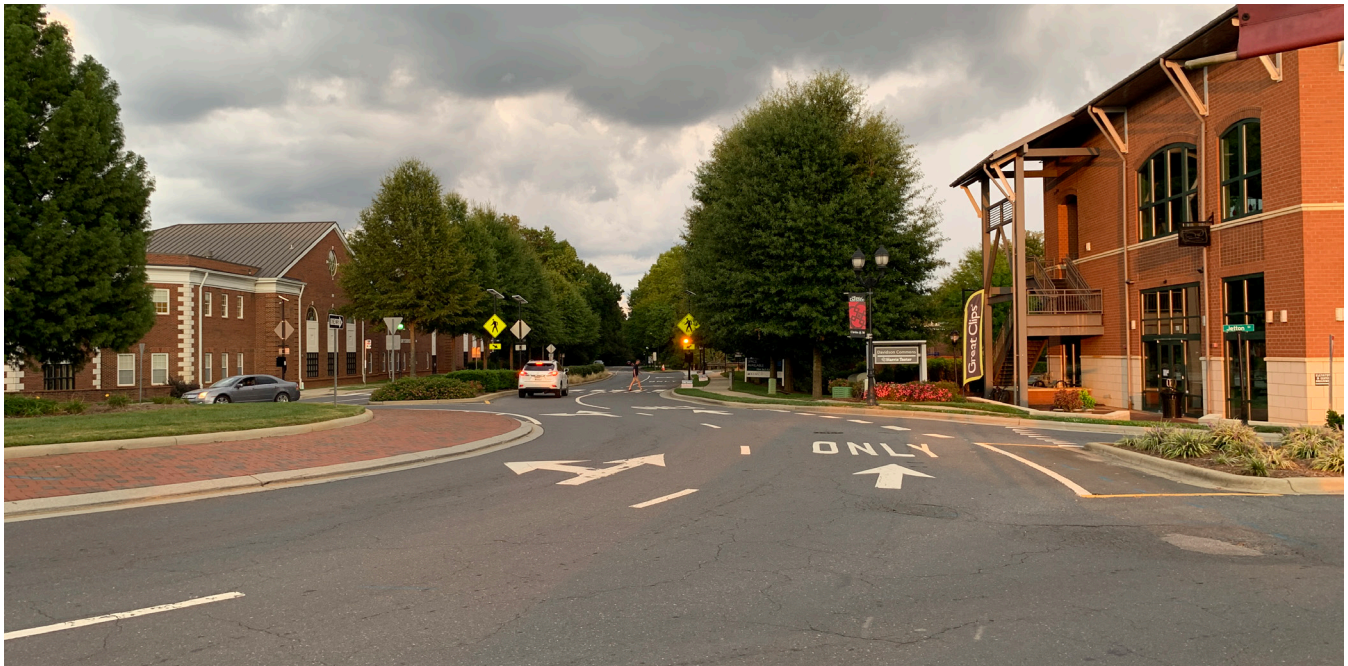
Figure 1. Multilane roundabout with RRFBs at pedestrian crossings. Source: FHWA.
