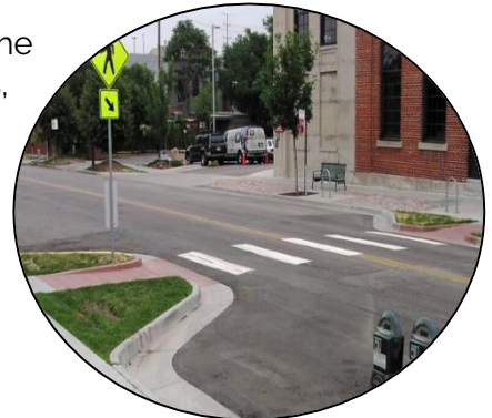
Curb extension example. Image Credit: Richard Drdul
