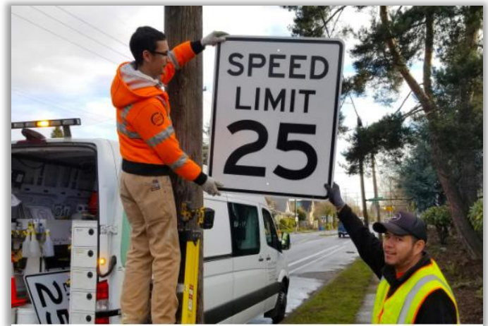
Workers replacing speed limit signs in Portland, OR. Photo Source: Portland.gov
