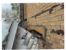
Existing repair failing due to age or improper repair.
