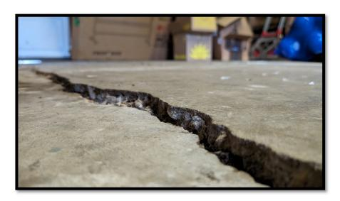
Figure 3: Garage S.O.G. Fracture
