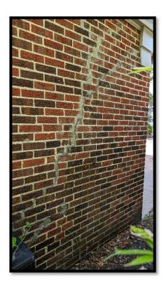
Figure 7: Foundation Settling Resulting in Brick Stair Stepping
