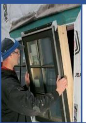
Windows with **Permanent Nailing Fins** require complete exterior window trim removal, and the windows must be installed on the outside. This results in a window being flush with the exterior wall giving it a non-historic appearance. Products that have removable nailing fins can be installed from the inside and are acceptable; only when the fins are removed, and the window is recessed within the opening.
