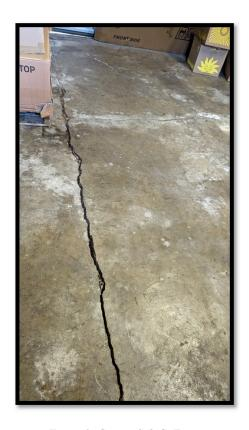
Figure 2: Garage S.O.G. Fracture
