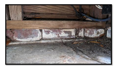
Figure 5: Garage Compromised (Non-Structural) Brick Curb
