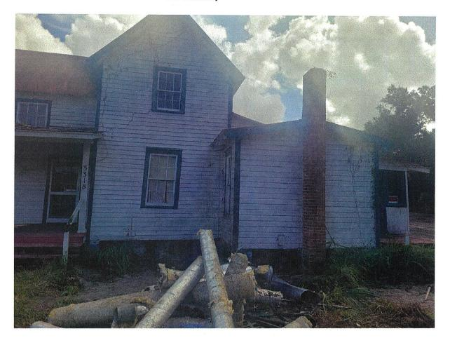
Photo 2 – Exterior of House on Brick Piers With Chimney Removed
