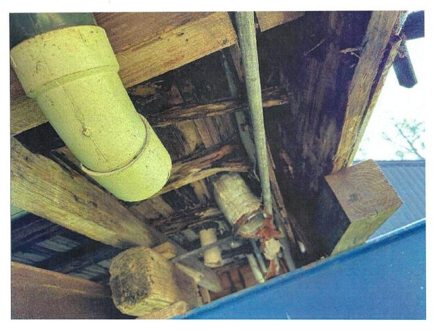
Photo 5 – House on Frame Showing Wood Frame Shoring/Repair
