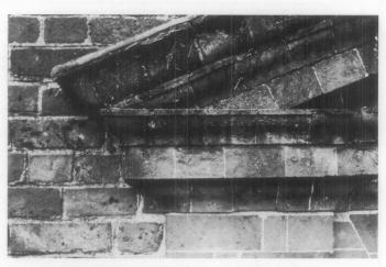
Figure 19. Mortar joints of 18th century brick buildings were often as much as 1/2 inch wide, cut flush and struck with a grapevine joint, but for window and door surrounds where a finer quality rubbed brick was used, mortar joints were very thin. Photo: National Park Service Files.
