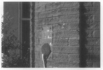
Figure 19. A comparison of undamaged bricks surroundng the electrical conduit with the rest of the brick facade emphasizes the severity of the erosion caused by sandblasting.
