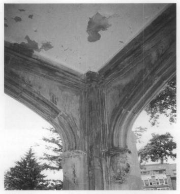
Figure 5. Repeated water washing did not remove the staining inside this limestone porte cochere. Upon closer examination, it was determined to be a water-repellent coating that had been applied many years earlier. An alkaline cleaner may be effective in removing it.
