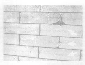
Figure 11. Rinsing with high-pressure water following chemical cleaning has left a horizontal line of abrasion across the bricks on this late-19th century row house.
