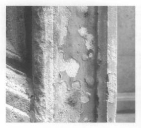
Figure 25. The clear coating applied to this limestone molding has failed and is taking off some of the stone surface as it peels. Photo: Frances Gale.
