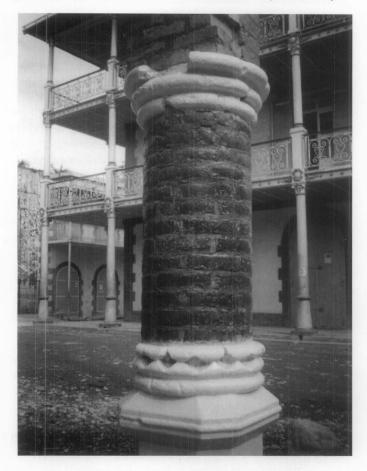
beneath the surface as subflorescence. Subflorescence eventually may cause the surface of the masonry to spall, particularly if a water-repellent coating has been applied which tends to reduce the flow of moisture out from the subsurface of the masonry. Although many of the newer water-repellent products are more breathable than their predecessors, they can be especially damaging if applied to masonry that contains salts, because they limit the flow of moisture through masonry.
