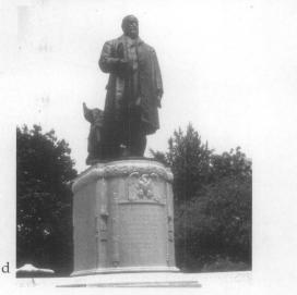
Figure 16. (a) The limestone base was heavily stained by runoff from the bronze statue above. (b) A poultice consisting of copper stain remover and ammonia mixed with fuller's earth was applied to the stone base and covered with plastic sheeting to keep it from drying out too quickly. (c) As the poultice dried, it pulled the stain out of the stone. (d) The poultice residue was removed carefully from the stone surface with wooden scrapers and the stone was rinsed with water. Photos: John Dugger.
