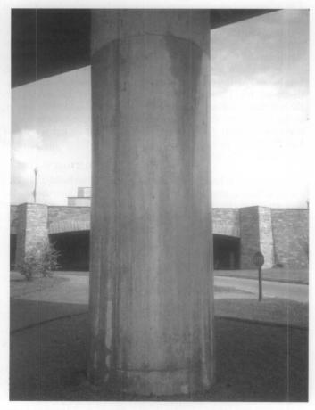
Figure 26. The anti-graffiti or barrier coating on this column is very shiny and would not be appropriate to use on a historic masonry building. The coating has discolored as it has aged and whitish streaks reveal areas of bare concrete where the coating was incompletely applied.
