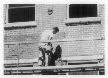
Figure 17. This photograph shows the significant visual change to the character of this historic brick building that has resulted from improper repointing procedures and a noticeably increased thickness of the mortar joints. Photo: Lee H. Nelson, FAIA. 359
