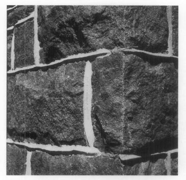
Figure 15. The profile of the repointed joints on the left replicate the historic joints around the corner to the right on the front of this stone building in Leesburg, VA. The contractor's pride in the repointing work is evident by the signature in the vertical joint. Photo: Anne Grimmer.
