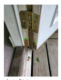
Wood decay fungus: Exterior 12) Damage to portions of rear French doors core & door jam.
