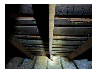
Drywood termite: Attic 17) Evidence of frass & damage to portions of roof deck boards rear right side.
