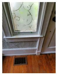
Wood decay fungus: Interior 13) Damage to portions of windows trim window right of front door.
