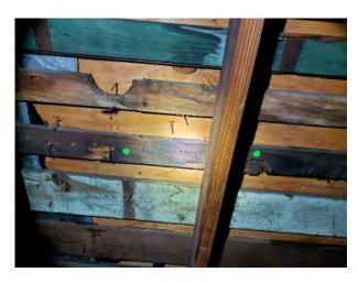
Drywood termite: Attic 16) Evidence of frass & damage to portions of roof deck boards rear left side.
