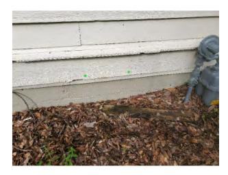
Wood decay fungus: Exterior 7) Damage to portions of lower trim right side near gas meter.
