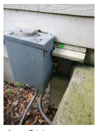
Wood decay fungus: Exterior 8) Damage to portions of trim rear of home behind ac unit.
