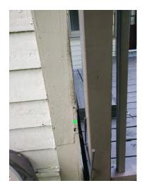
Wood decay fungus: Exterior 9) Damage to portions of trim corner back right of back deck.
