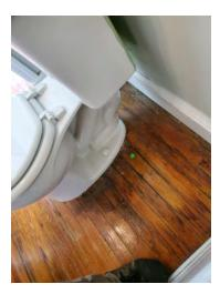
Wood decay fungus: Interior 14) Damage to portions of floor at toilet first floor rear right bathroom.
