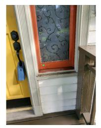
Wood decay fungus: Exterior 5) Damage to portions of windows trim right of front door.
