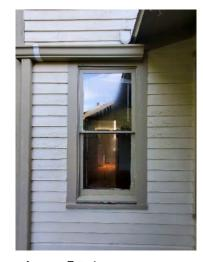
Wood decay fungus: Exterior 10) Damage to portions of upper & lower windows trim & sill middle window between back doors.
