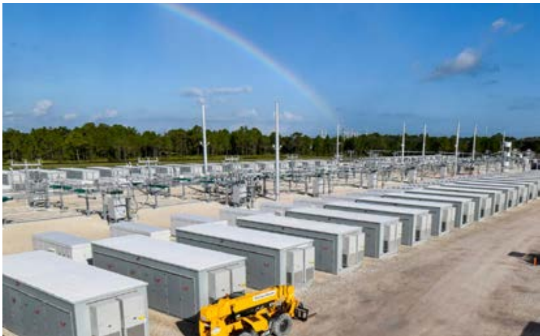
FPL- Battery enclosures at Manatee Energy Storage Center, hailed by FPL as the world’s largest solar-charged BESS when it went into operation in 2021.
