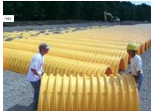
Figure 7 Installation of corrugated arch system. Figures courtesy of the following companies: ACF Environmental, Contech, GeoStorage, ITS, Raintank. Image 10 of 17
