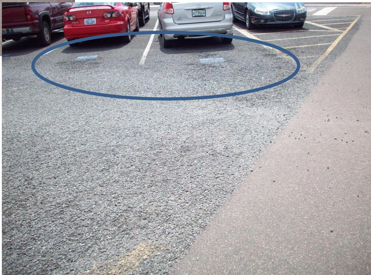
Solution: thin standard asphalt drive aisle and auto pivot points,
