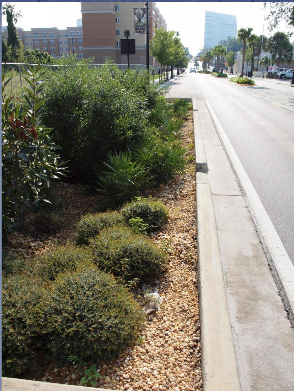
Bioswale Stormwater Treatment
