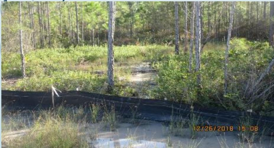
DEP Manual points out that black fabric does not protect against turbidity – recommends *double row* of silt fence and other turbidity controls
