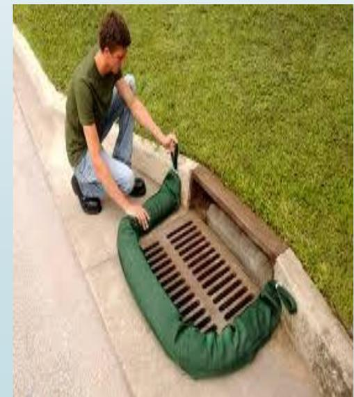
Diversion, wrap, sandbag, etc. The DEP Manual gives details on appropriateness and installation of different BMPs.
