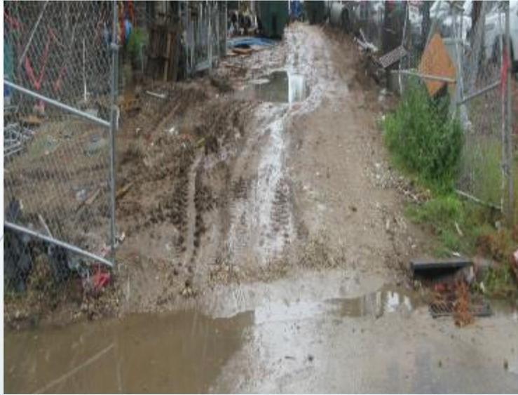
Stabilization to prevent track out is outlined with specificity in the manual. Track out is one of the largest contributors to unlawful discharges to stormwater. There are also reusable technologies available such as fods, rumble strips, etc.
