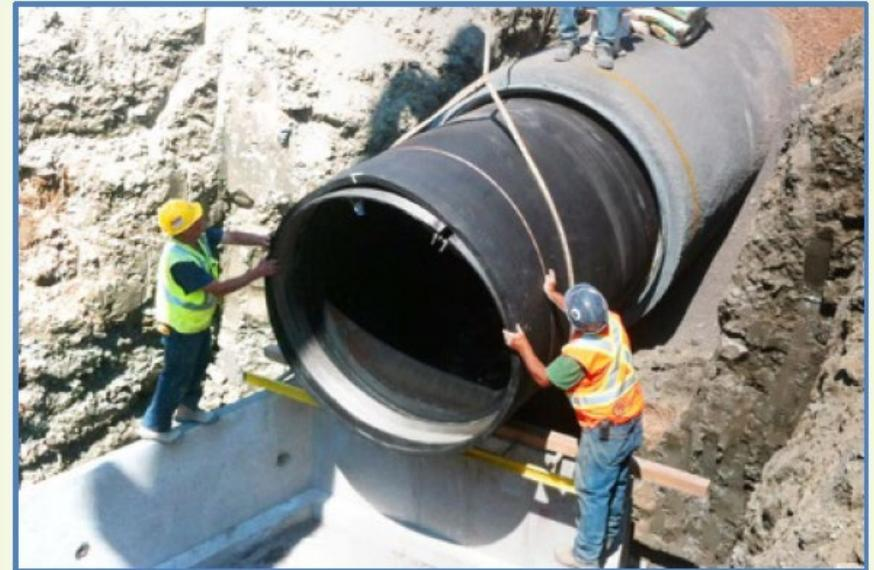
One type of tide check valve, Tideflex CheckMate Inline Check Valve<sup>[6]</sup> will allow stormwater to drain out under lower tide conditions. During high tide, the valve will prevent sea water from backing up into the stormwater pipe network.
