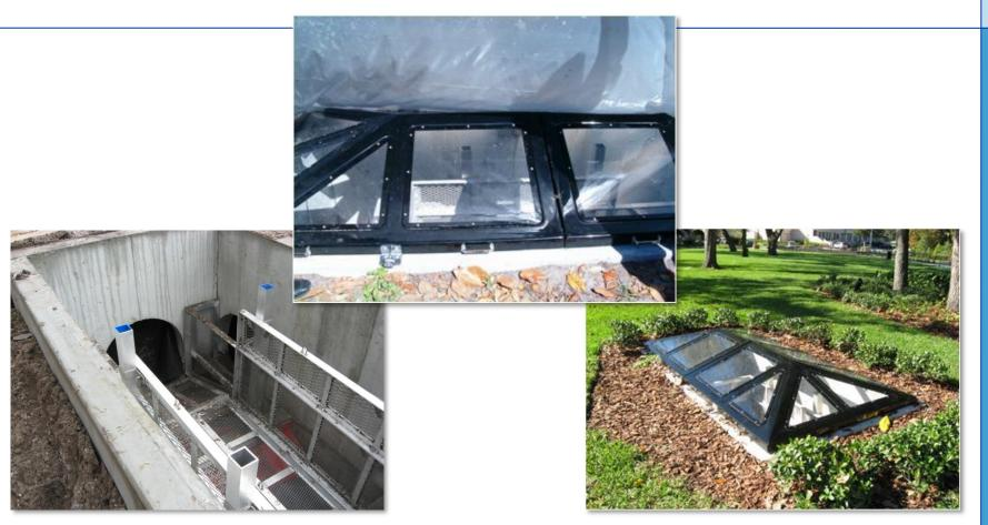
Baffle box with viewing cover allows visitors to see the mechanics behind an otherwise invisible technology
