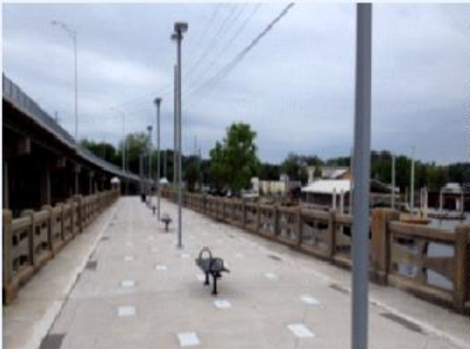
Trout River Pier; Photo provided by Brian Burket, Jax Parks
