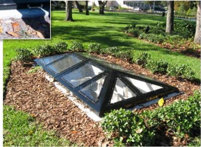
**Baffle box with viewing cover allows visitors to see the mechanics behind an otherwise invisible technology**
